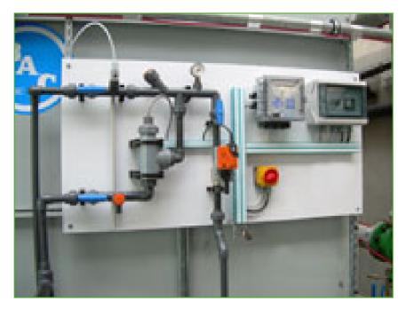
BAC offers a wide range of **automatic water treatment packages** to control corrosion, scaling, fouling and microbiological growth in cooling systems incorporating BAC closed circuit coolers.
