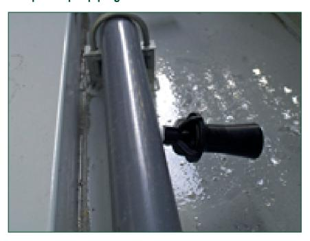
A sump sweeper piping system **increases water circulation and agitation in** the basin and is designed to be used in combination with a **filtration** system. It does all this:
